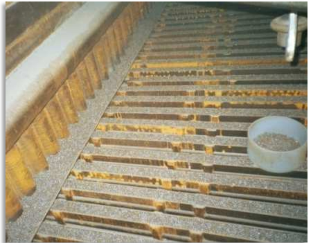
Arrangement of tube protection
